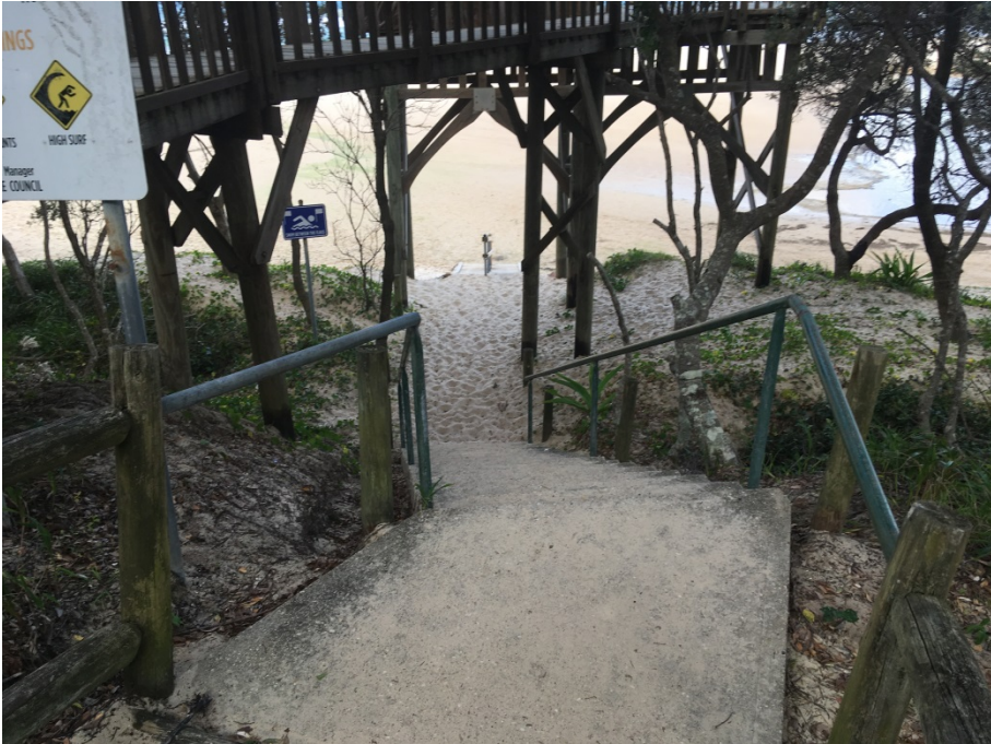
Plate 2. Pedestrian access stairs running under the USLSC lookout tower (looking south east)
