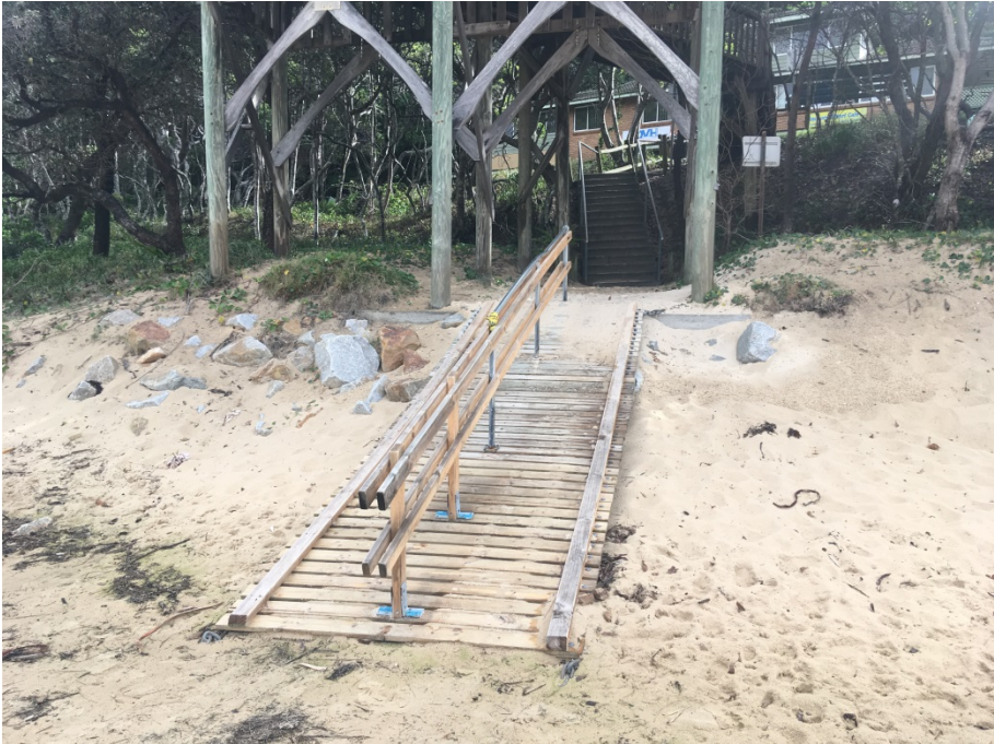
Plate 3. Temporary access ramp for pedestrians under USLSC lookout tower (looking west)
