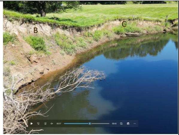
Plate 4 Looking downstream at Section B/C
