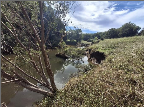
Photo 3: Overview of the upstream section of the Riverbank works Date: 20/3/2025
