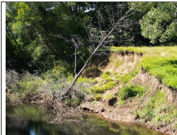
Plate 1 Looking upstream at Section A – relatively stable profile
