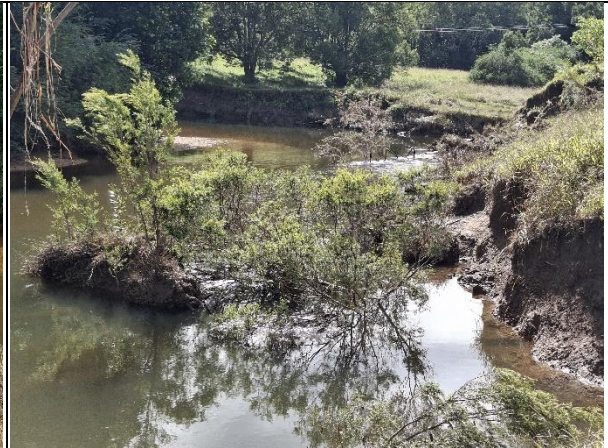
Photo 2: Overview of the midstream section of the Riverbank works Date: 20/3/2025
