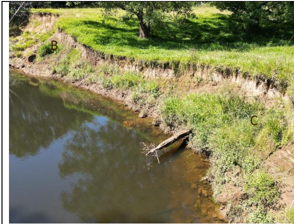
Plate 3 Looking upstream at Section B/C
