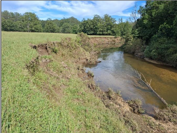
Photo 1: Overview of the downstream section of the Riverbank works Date: 20/3/2025
