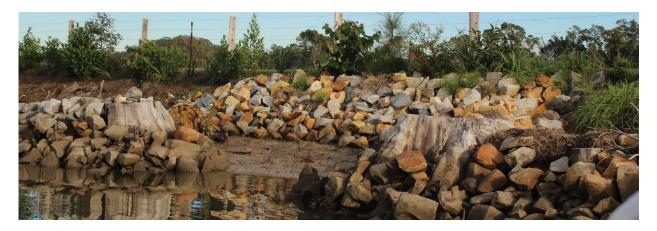
Figure 29. Rock fillet bank stabilisation works recently implemented in Kalang River lower estuary
