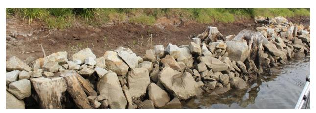
**Figure 30.** Rock fillet bank stabilisation works recently implemented in Kalang River lower estuary
