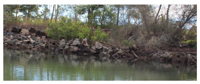
Figure 31. Fish ball and rock fillet bank stabilisation works recently implemented in Bellinger River lower estuary
