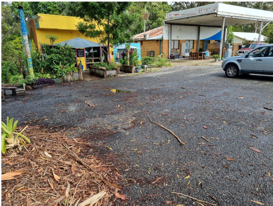
Figure 1: Liberty Providores cafe - yellow building
