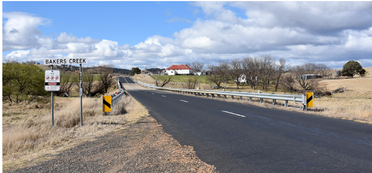
Safety improvement work to start at Bakers Creek
