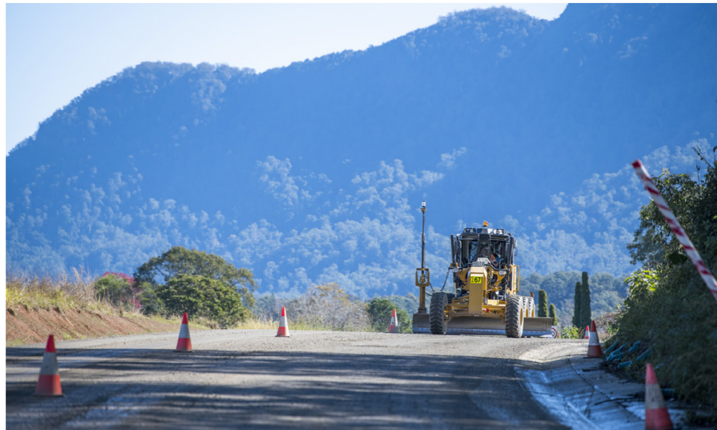
Grader at work, Pump Station to Fernridge Lane
