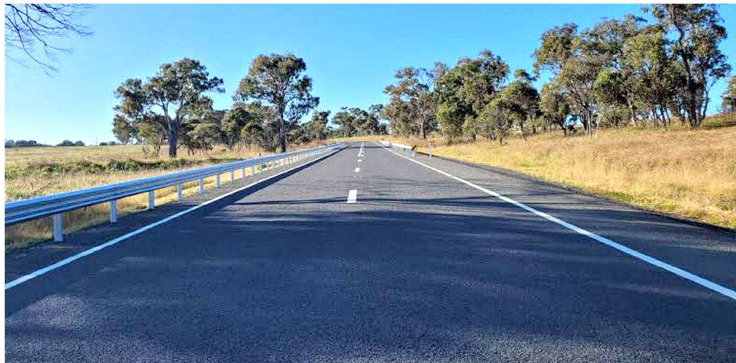
Work completed at Sandy Creek to Wakefield Road
