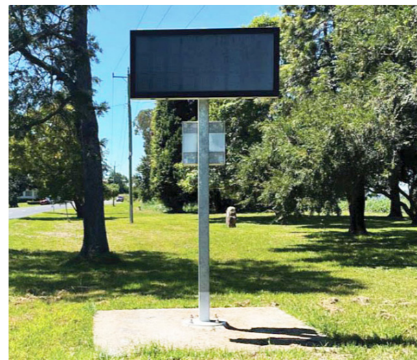
Example of variable message sign to be installed
