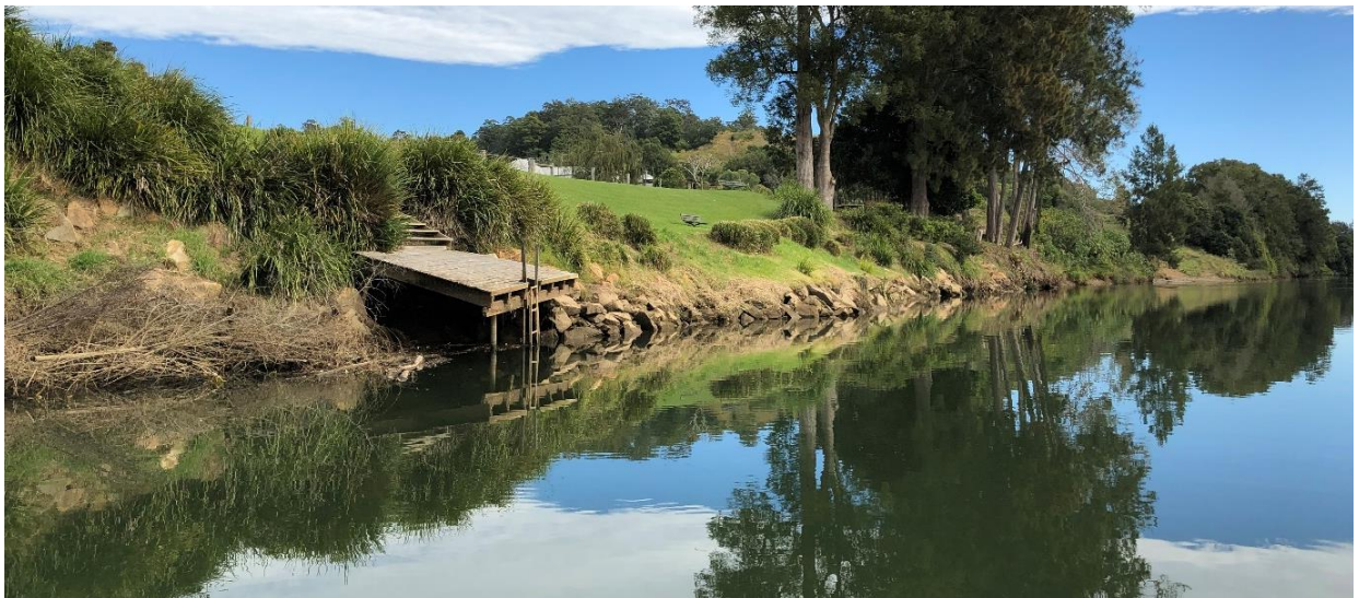
Figure 28. Historic bank stabilisation works to protect a landholder pontoon within Bellinger River upper estuary
