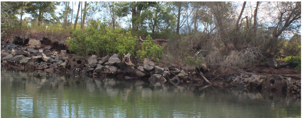
Figure 31. Fish ball and rock fillet bank stabilisation works recently implemented in Bellinger River lower estuary
