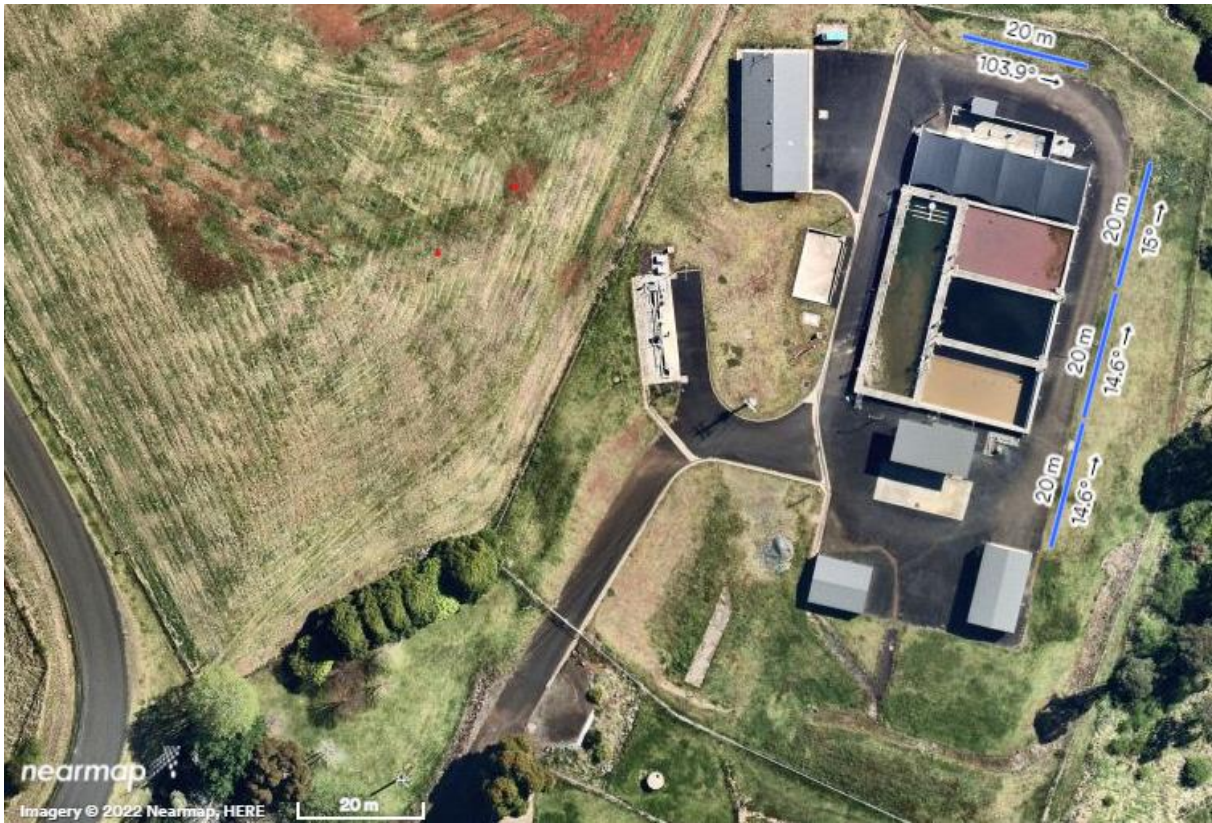
Figure 6-2 Location of Dorrigo trial at Dorrigo Sewage Treatment Plant.
