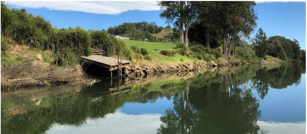
**Figure 28.** Historic bank stabilisation works to protect a landholder pontoon within Bellinger River upper estuary
