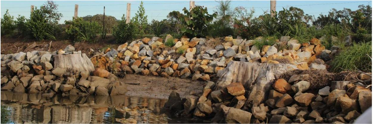
**Figure 29.** *Rock fillet bank stabilisation works recently implemented in Kalang River lower estuary*
