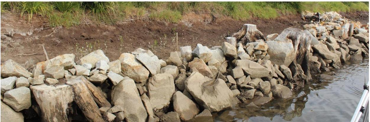
**Figure 30.** *Rock fillet bank stabilisation works recently implemented in Kalang River lower estuary*
