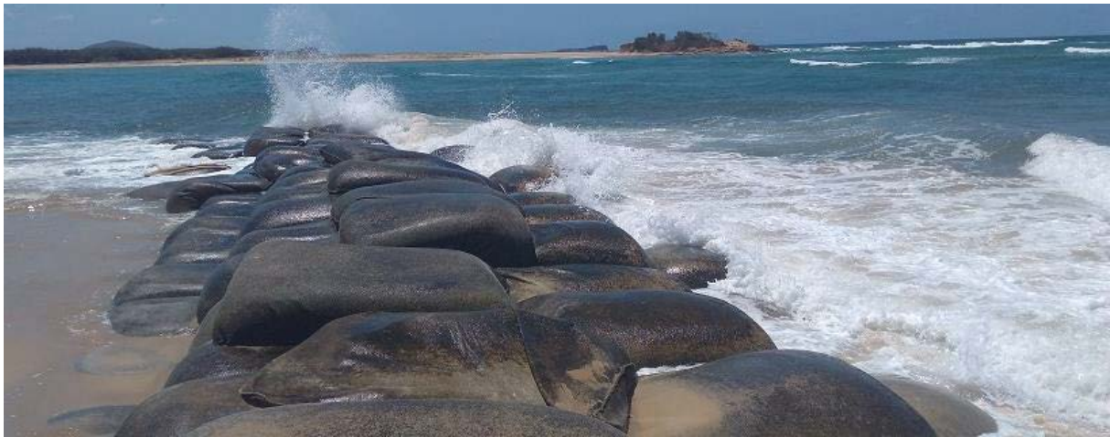
Plate 2. GSCs used for coastal groyne construction (JBP 2017)
