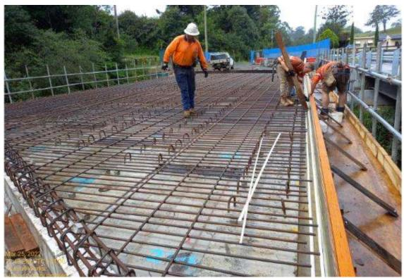
Concrete deck pour with elevated walkway attached to bridge planks
