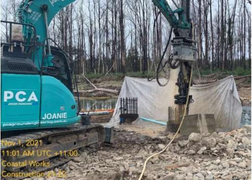
Excavator mounted rock anchor drilling setup (7-12t sized machine) with splatter screens used next to waterway
