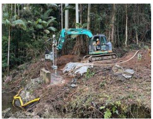
Same smaller excavator (7t) rock anchor rig
