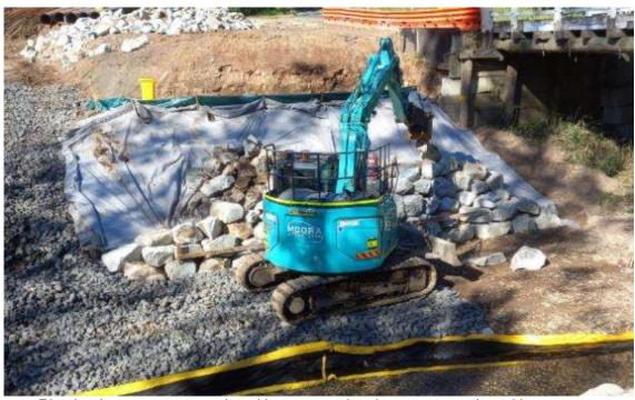
Riverbank access ramp and working area and rock scour protection with excavator
