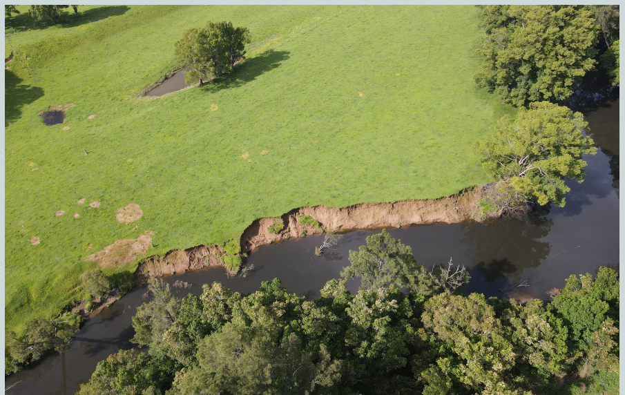
Aerial and drone photography allowed the project team to inspect the extent of issues such as riverbank erosion.
