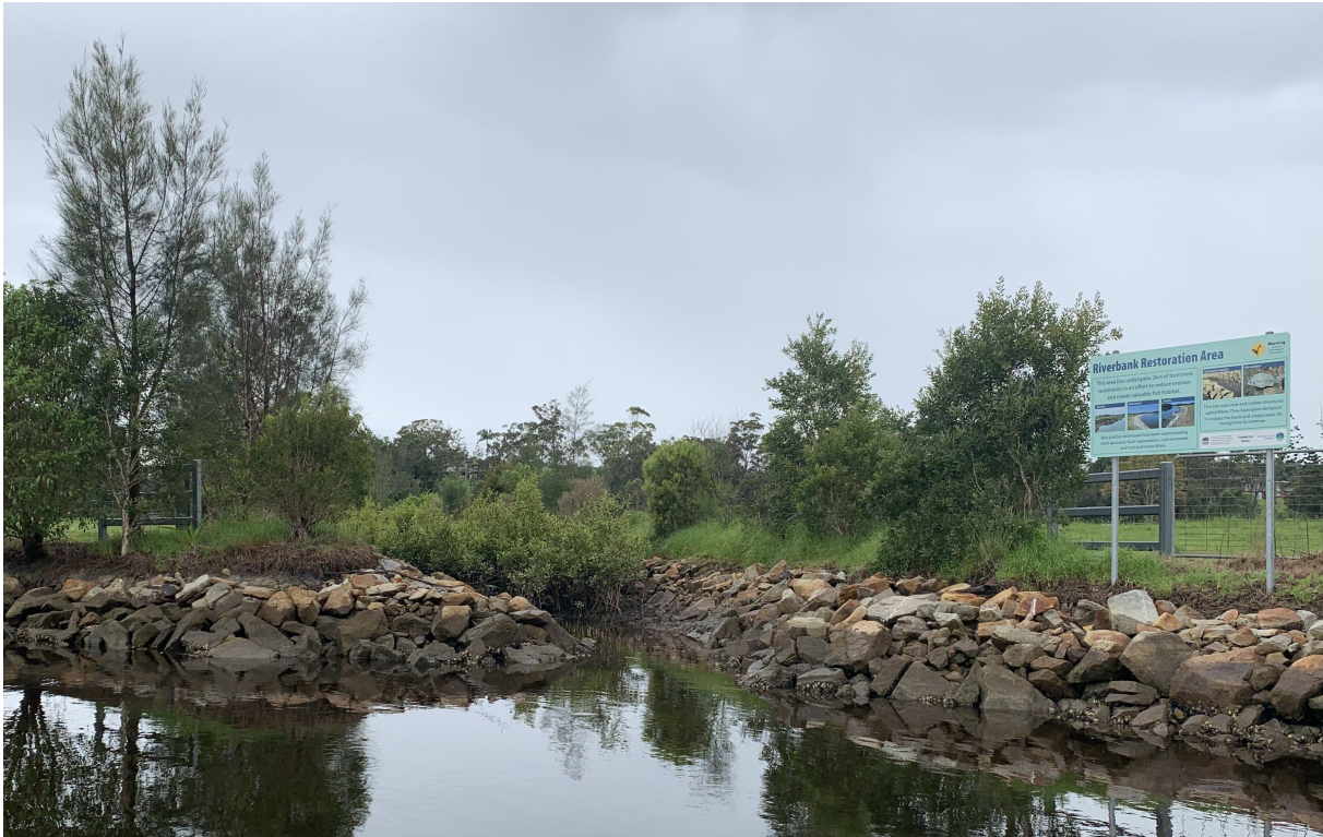
Figure A-24 Mangrove re-establishment following stabilisation of drainage line, Newry Island
