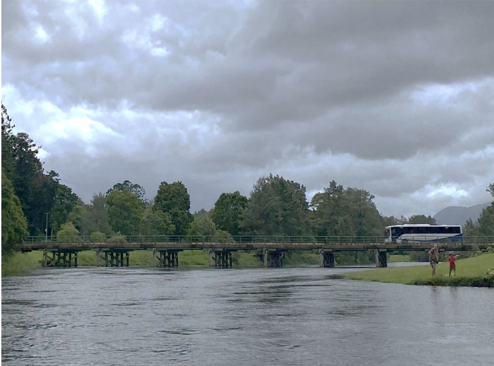
Figure A-3 Lavender Bridge at Bellingham, near Tidal Limit of Bellingham River (captured High Tide, 6 December 2021)
