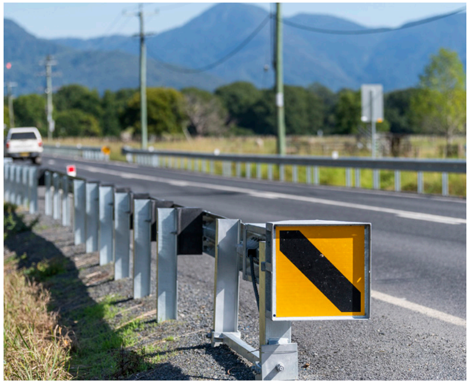
Newly installed guardrail, east of Bellingen
