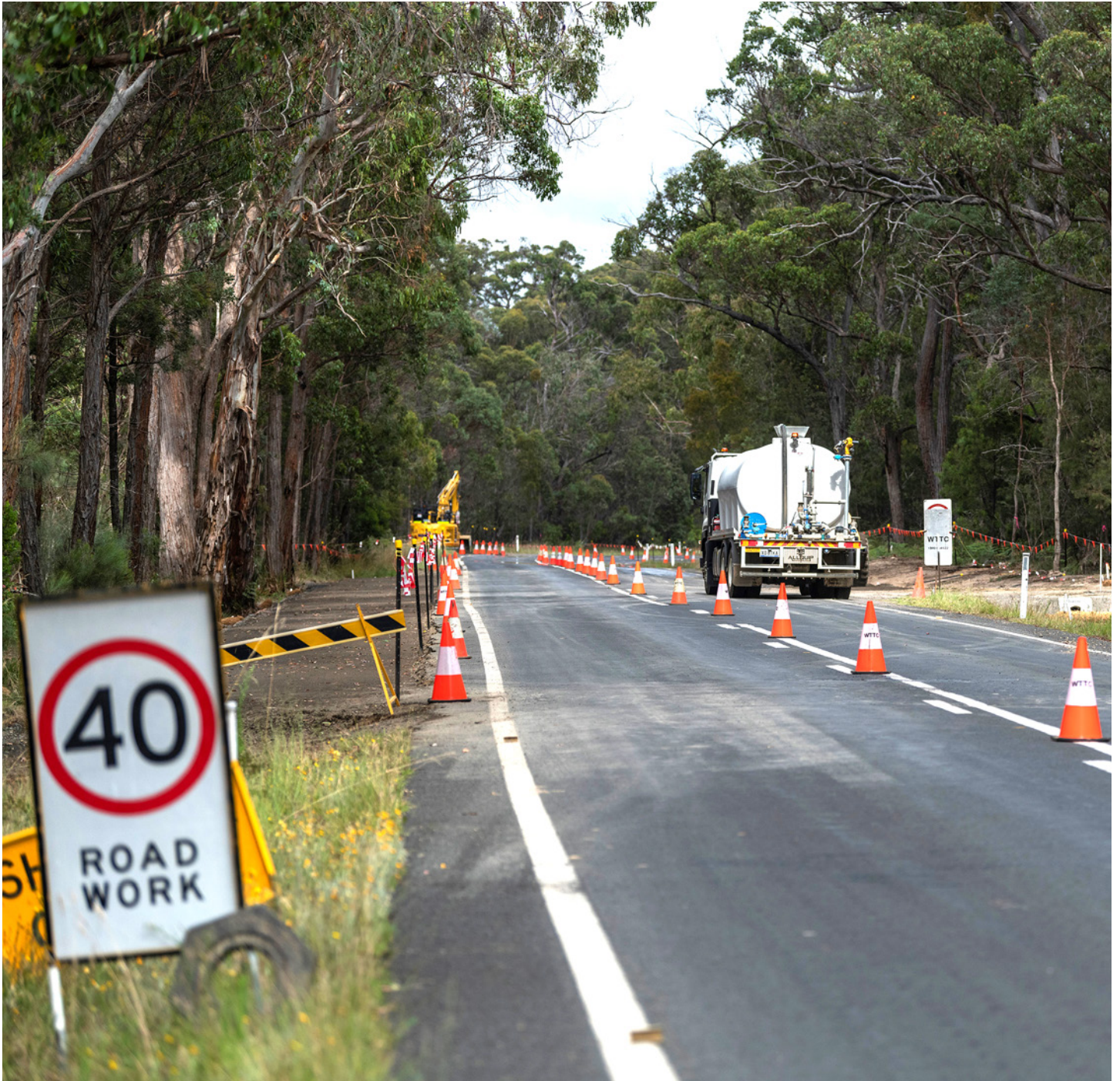
Ongoing construction work, Appledale to Scotsburn*, east of Armidale
