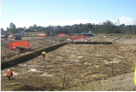
Excavation to biofilter base
