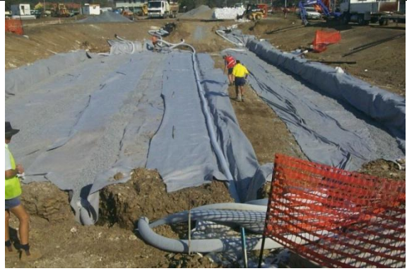
Placement of underdrains and impermeable liner
