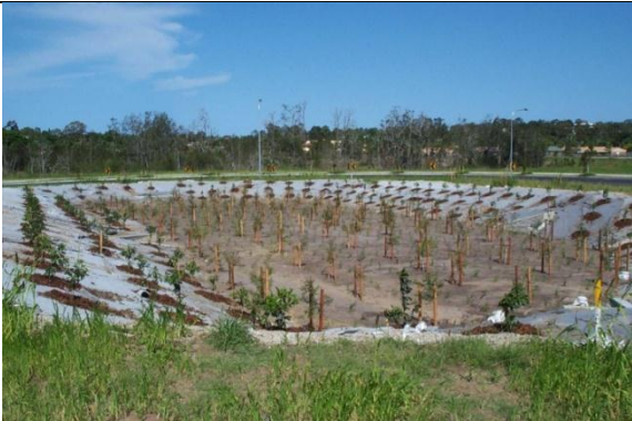
Biofilter planting completed
