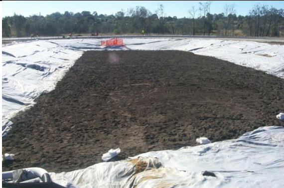
Biofilter media placed
