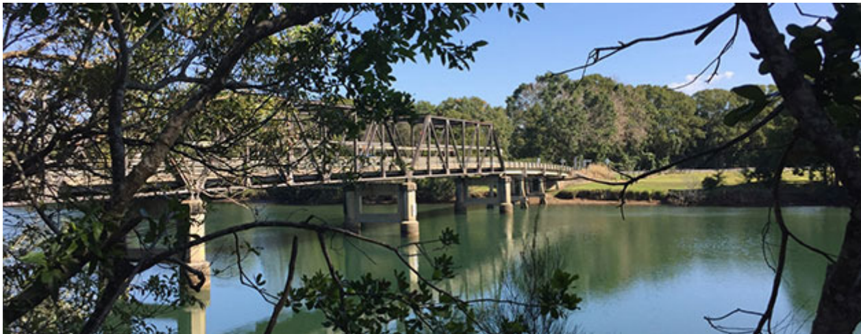
Raleigh Bridge over the Bellingier River
